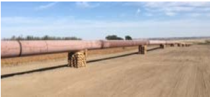
(Pipe strung up, welded and waiting to be pulled under canal when drilling is finished)
